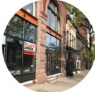
Ground floor commercial space
