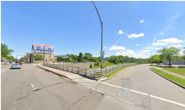
The intersection of North Street and Delevan Street, overlooking the Inner Loop, lacks quality streetscape/urban design features and does not promote safe or comfortable access to parks Source: Google Maps
