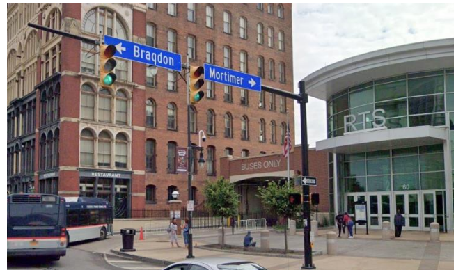
The RTS Transit Center on Mortimer Street Source: Google Maps
